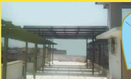
Raised Rooftop installation
